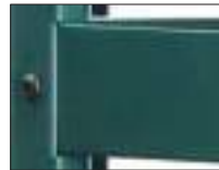
Column with folded edge for increased support for the middle tray
